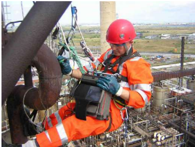
A worker inspecting a pipe by industrial radiography testing
